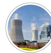
Thermal Power Generation
